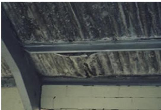
Damaged asbestos cement roof
