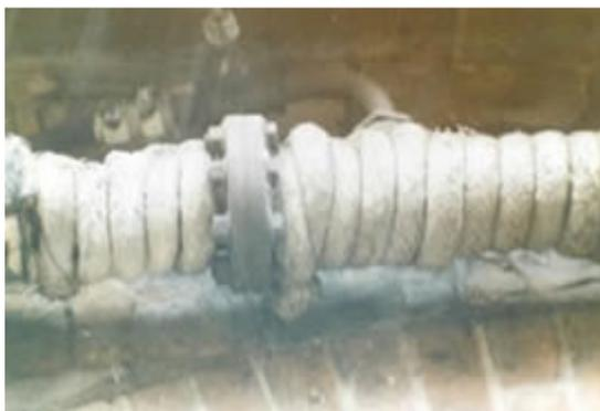
Asbestos rope used as insulation on a pipe
