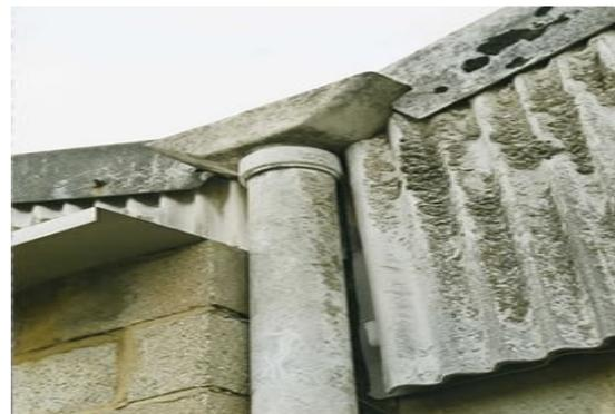
Asbestos cement downpipe, hopper and profile sheet
