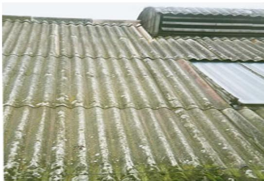
Asbestos cement roof (weathered exterior)
