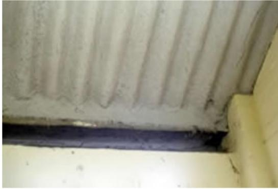
Sprayed 'limpet' asbestos on the underside of an asbestos cement roof
