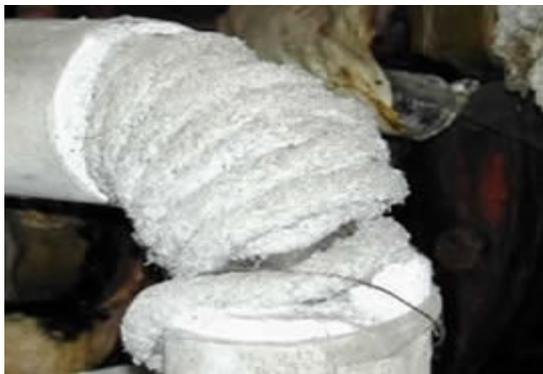
Pipe insulated using both asbestos lagging and rope
