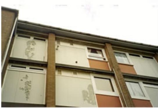
Damaged asbestos panelling
