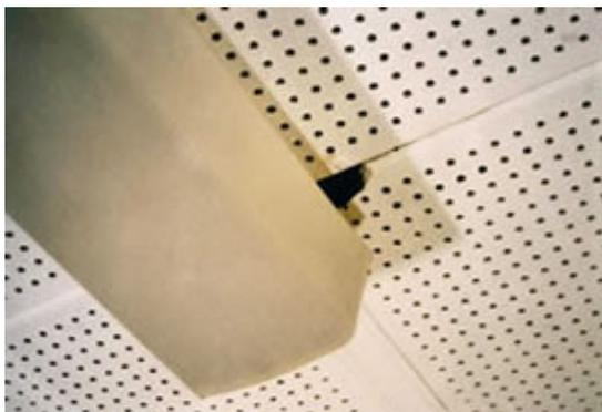
Perforated AIB ceiling tiles damaged around the light fitting
