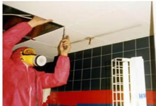
Unscrewing of an AIB ceiling tile
