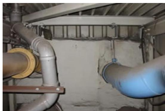
Wall with trowelled loose asbestos
