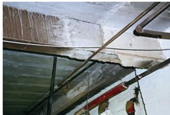
Sprayed 'limpet' asbestos coating which has been partly removed
