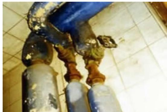
Damaged asbestos lagging on hot water pipes
