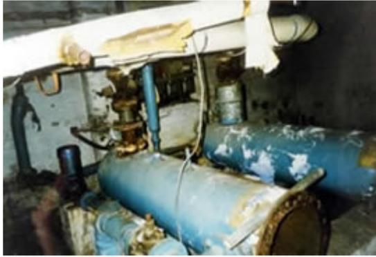
Damaged asbestos pipe lagging and debris
