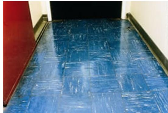
Asbestos containing vinyl floor tiles
