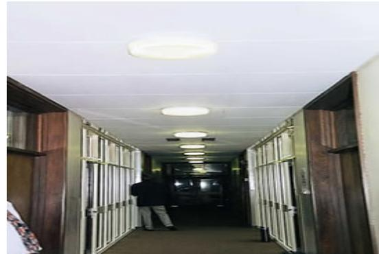
Suspended AIB ceiling tiles in a corridor
